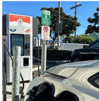
Public Parking Lot, CA USA
